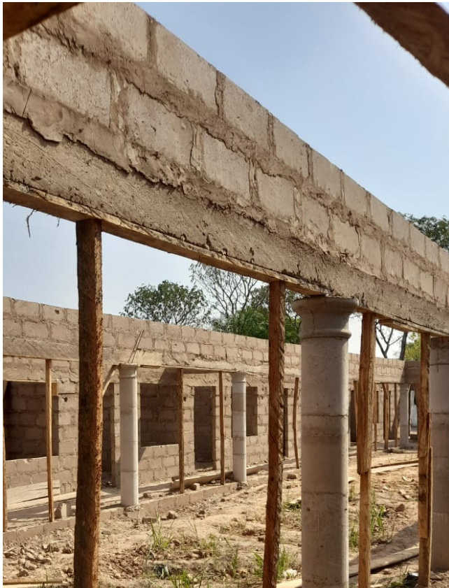
Dome Clinic under construction
