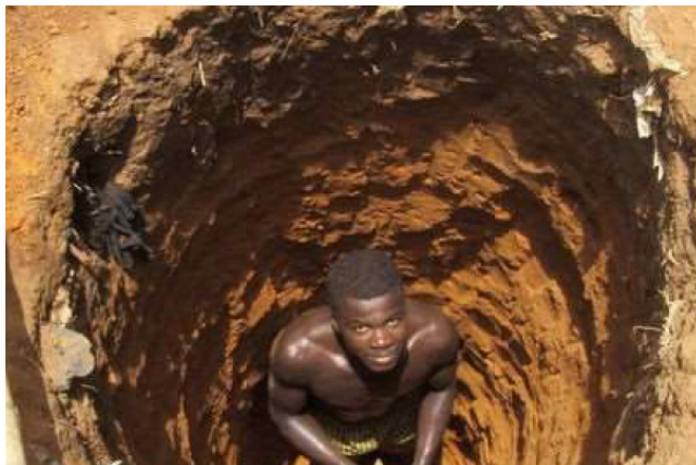
Digging a latrine pit
