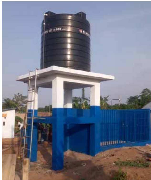
Overhead water tank
