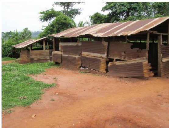
Existing traditional pit-latrine (building)
