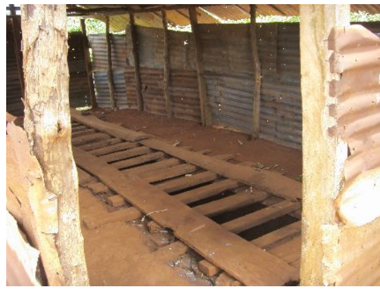
Existing traditional pit-latrine (seats)
